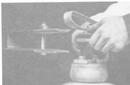
Figure 8 — Adjusting arcing horn.
